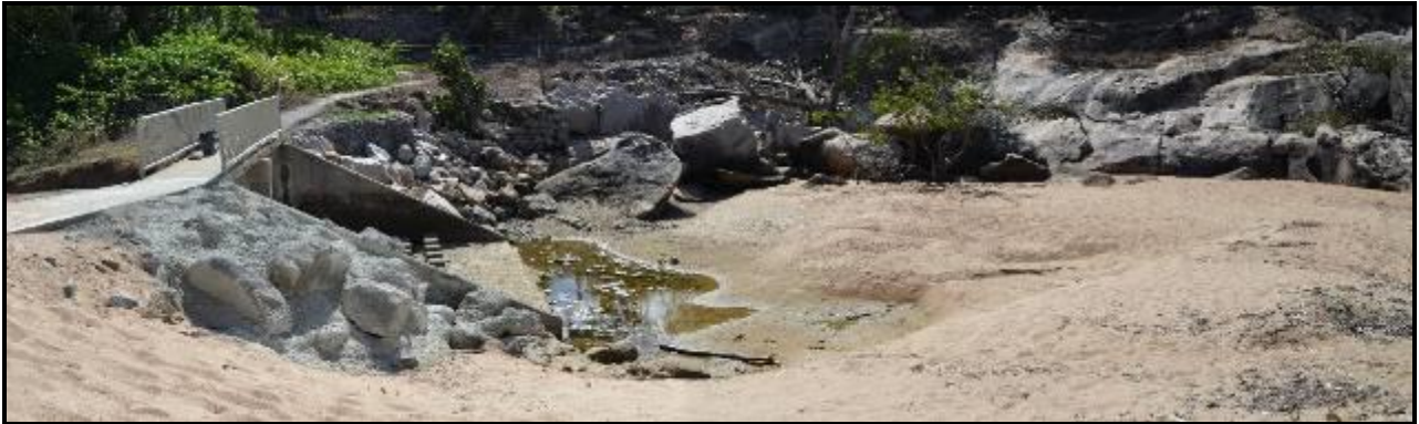
Figure 3-5 Alma Creek Footbridge
